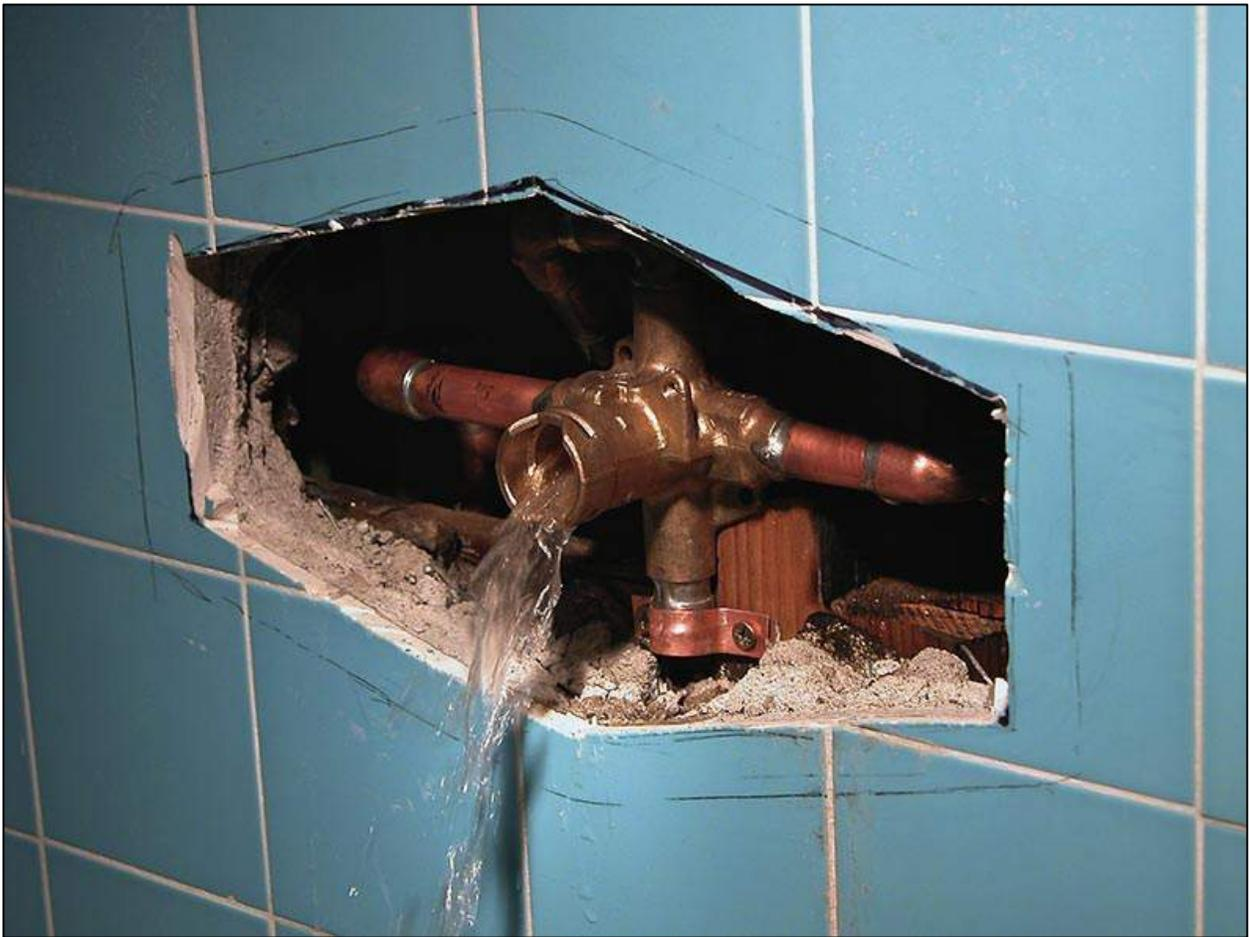
ALWAYS remove the Tub and Shower Valve Cartridge after installing a new valve and purge the in-wall valve!!! In California, building codes require Pressure Balancing Shower and Tub & Shower Valves. In short, this means if there is not equal pressure on the Hot and Cold sides of the valve, no water will come out and you won't be accidentally scalded by unexpected hot water.
