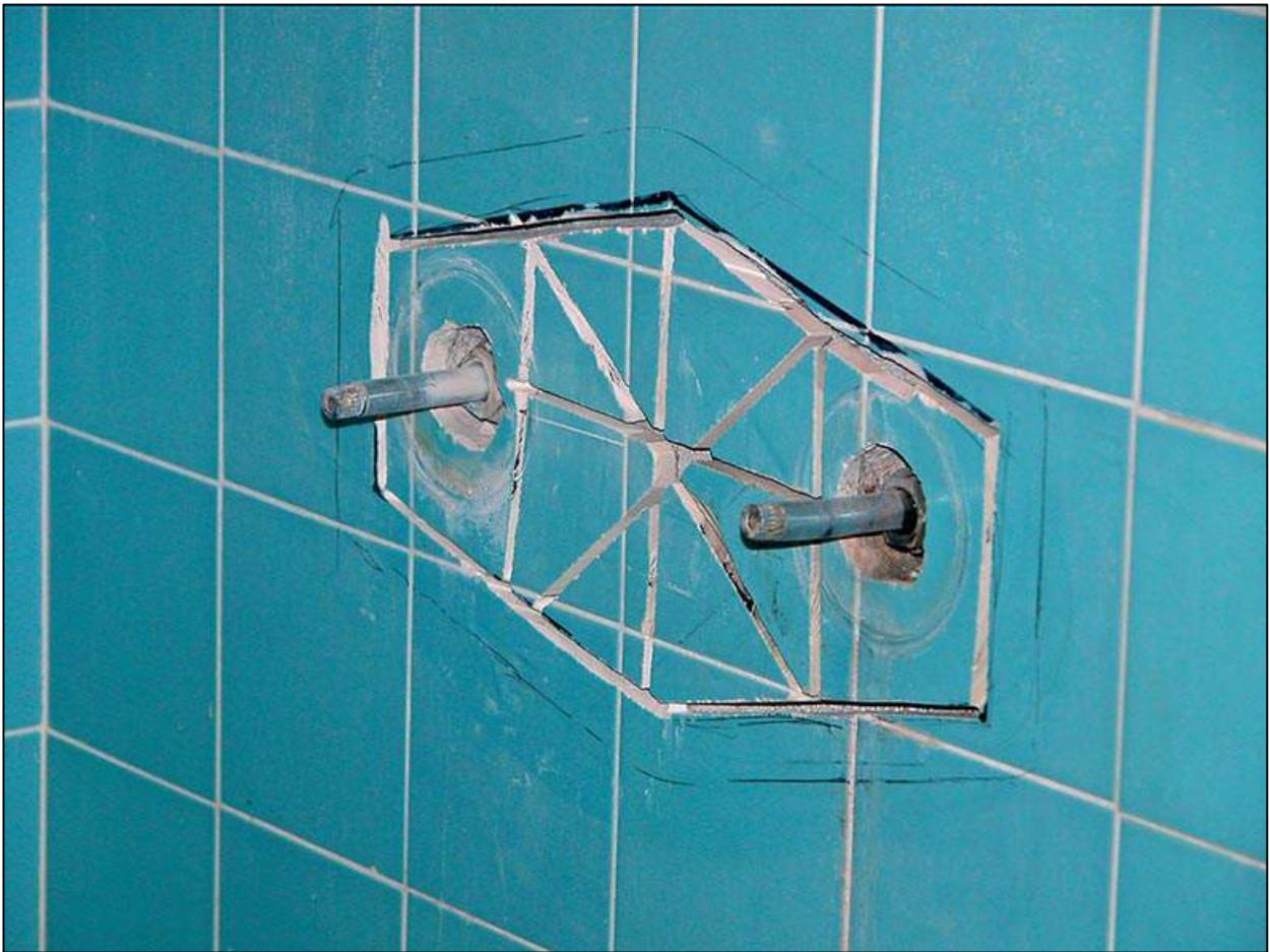
This photo shows the tile cuts and the various cross cuts to control the breaking of the tile and concrete wall float behind. Of course there's no 100% guarantee you will not lose a small tile piece during this process, but when doing control cuts, it's very rare that would happen.
