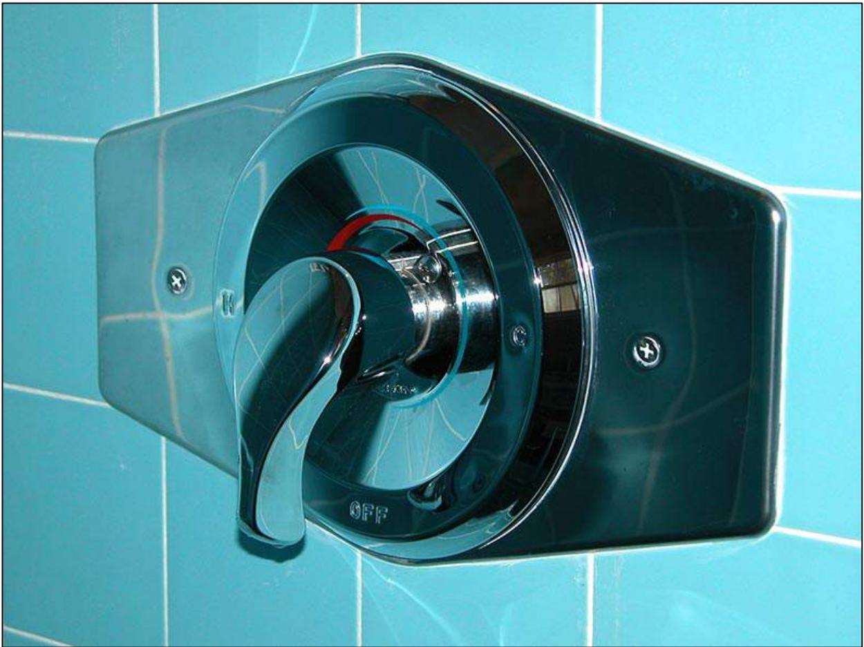
This final photo shows the Shower Valve with the Repair Plate, face plate, handle and fixtures installed. Also notice the water proofing sealant at the edges of the Repair Plate, faceplate, and even Phillips head retaining screws.
