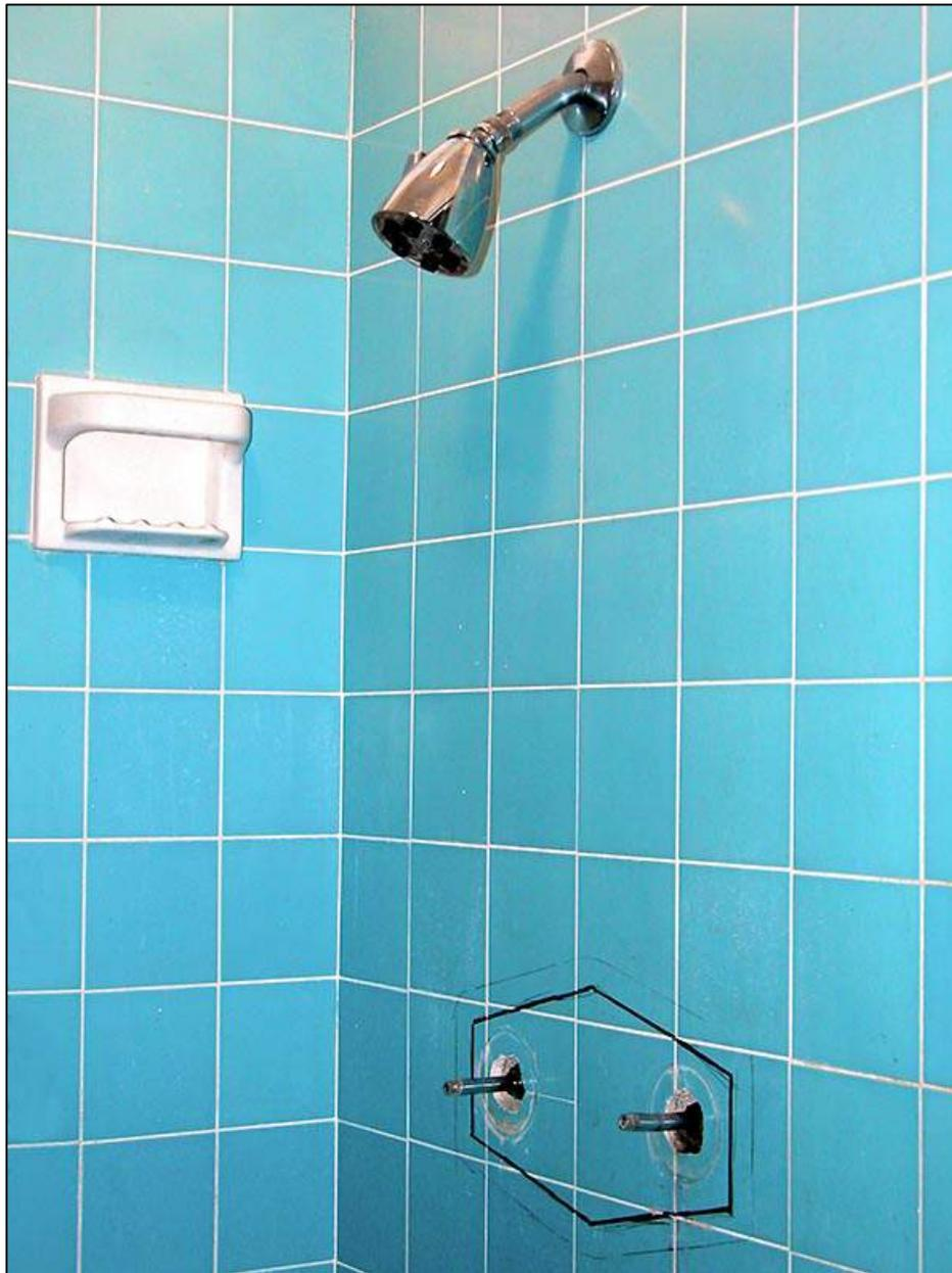
This original Shower Valve had stems and handles that could not be removed. As you can see, the Valve Stem on the right had to be broken to be removed. This customer was also in danger of flooding due to the lack of readily available rebuild parts.
