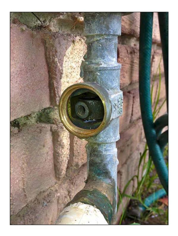
In the above photo you can see the Gate actually lodged in the body of the valve. Luckily we were able to disassemble the 'bonnet' (the part of the valve that holds the screw / stem assembly and handle) and remove the lodged Gate.
