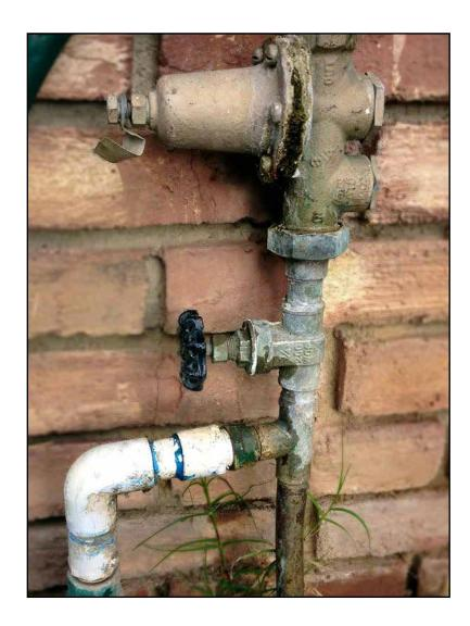
To temporarily get water to this house, we were able to assemble the valve (without the Gate of course) and turn the water back on. This is a very temporary solution. In case of a sudden break or natural disaster, you will need to immediately be able to turn the water off and on to your house!
