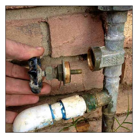
Because of their low price, Gate Valves are often installed in new homes and during repairs by handymen or plumbers that are trying to save a few dollars on material. The problem is, due to the nature of their design, they often fail.
